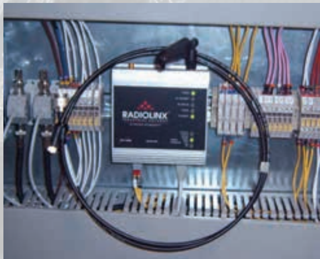
ProSoft Technology® radios operate as an automatic fallback connection, should the fiber optic connection be lost.
