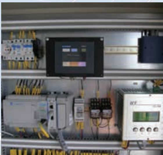
ProSoft’s IEC 60870-5-101 module for MicroLogix™ gathers data from a solar power plant’s photovoltaic process.
