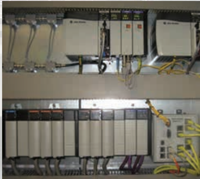
ProSoft Technology's PROFIBUS® module for ControlLogix® facilitates communication from drives in a flood defence system in Kent, England.
