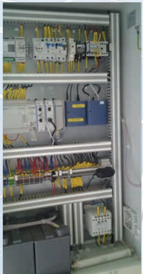
ProSoft’s IEC 60870-5-101 module for MicroLogix™ gathers data from a solar power plant’s photovoltaic process.
