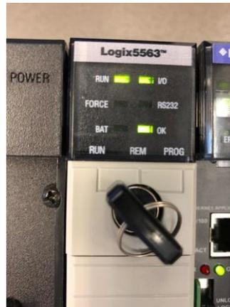
Key switch in RUN position – key removed:
